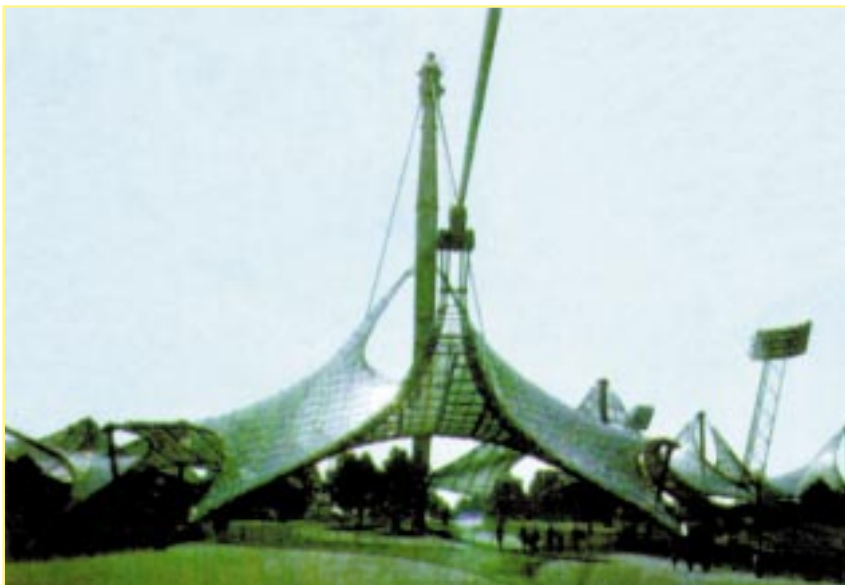
The roof of the Munich Olympic Stadium was inspired by spider webs. In this way the various tensions are evenly distributed over the roof.
